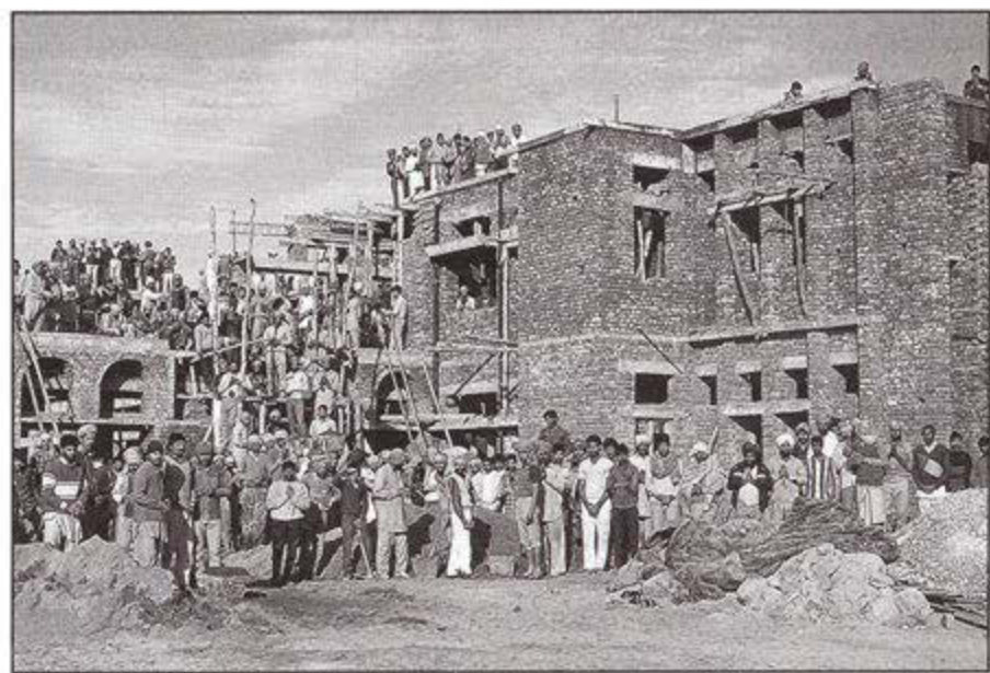
A large group of sevadars casting a roof slab.
