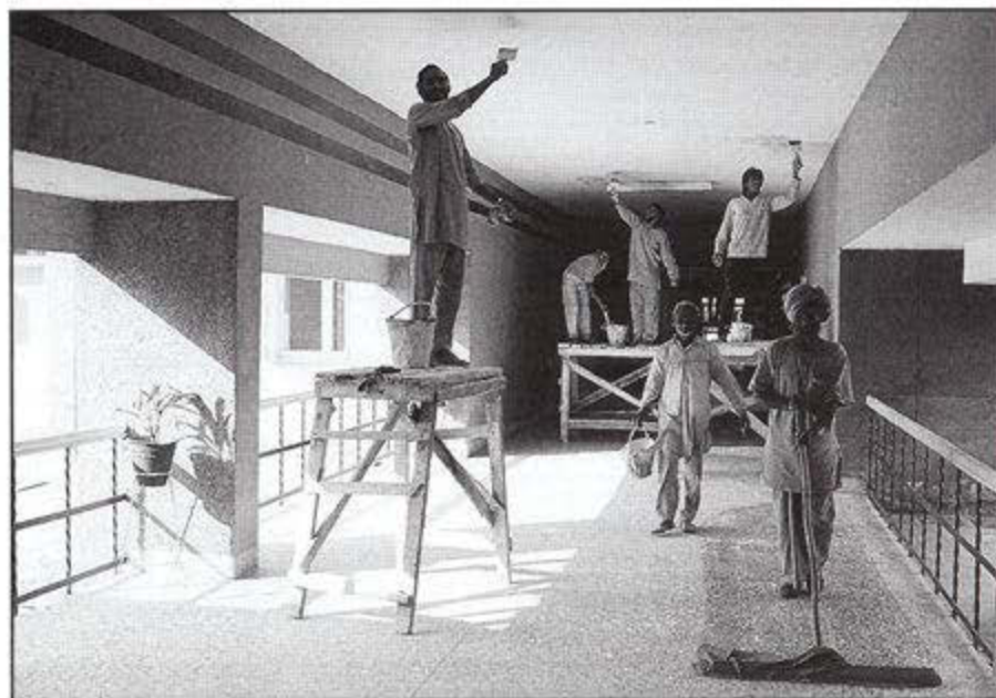
Sevadars with the Civil Maintenance Department painting the corridors.
