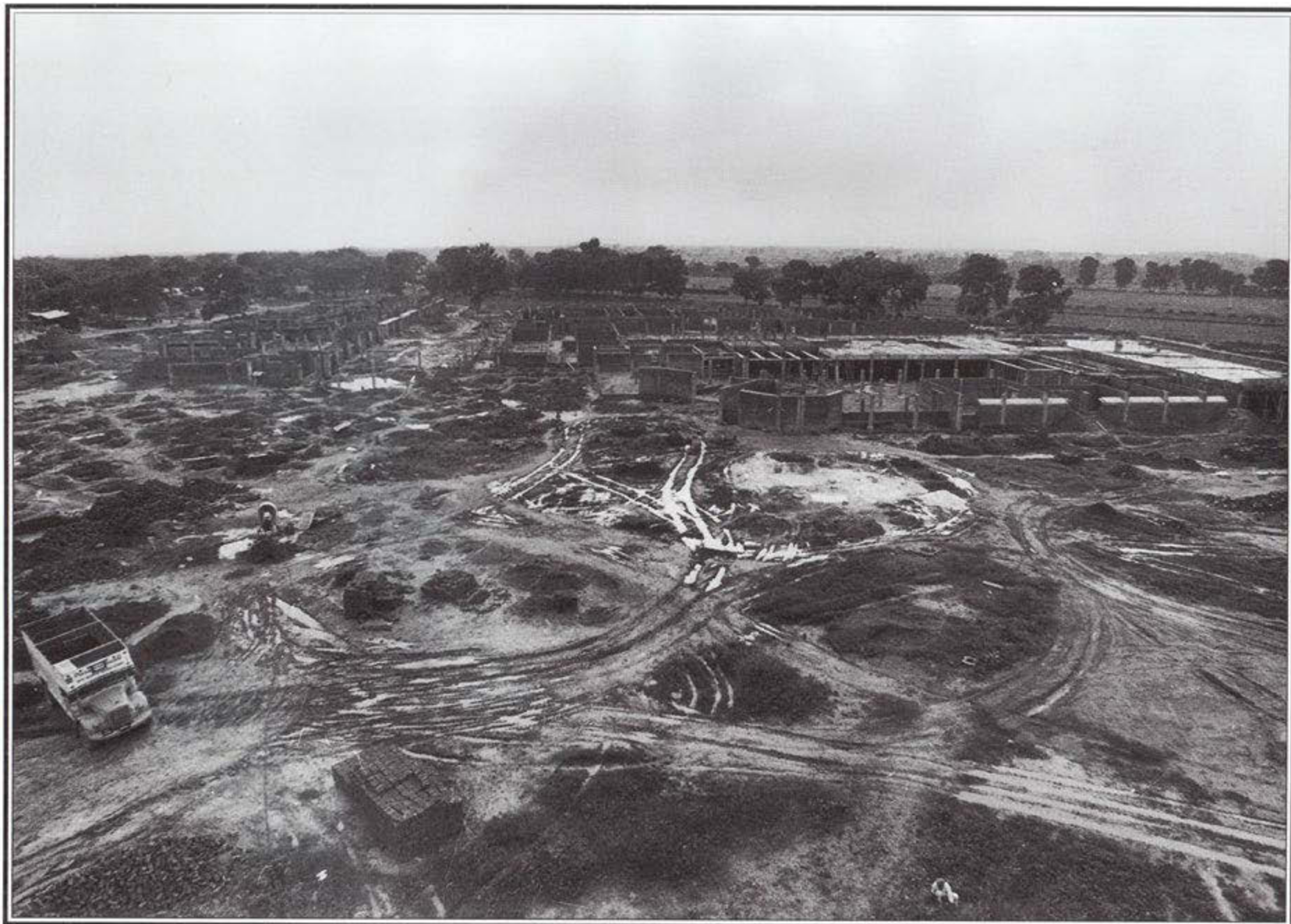
The hospital site during the early days of construction.
