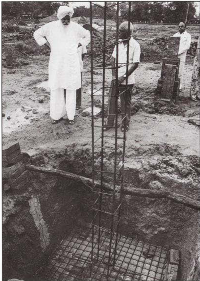
(Above) Inspecting a column and pier reinforcement. (Right) Various supply stores.
