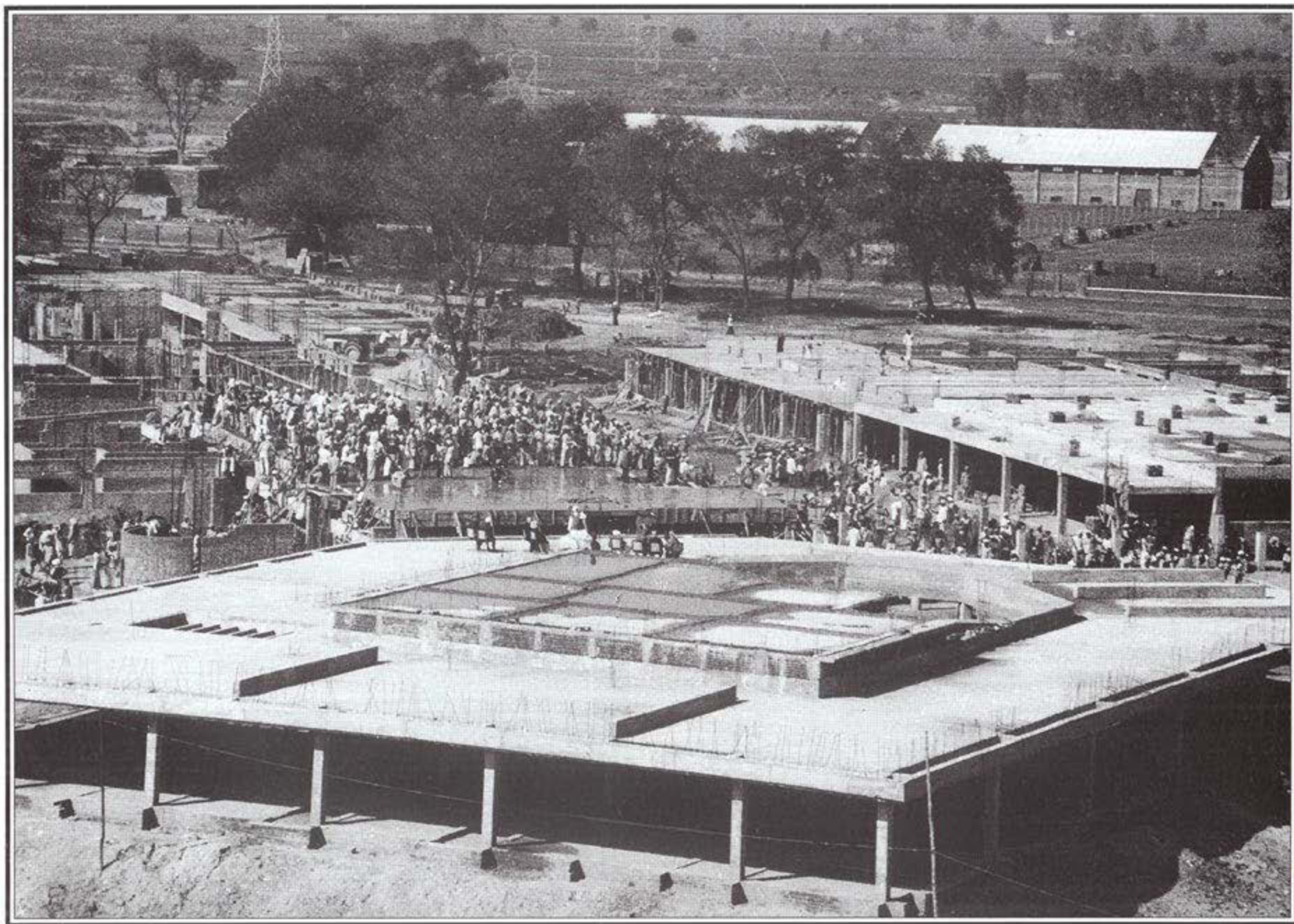
The casting of a roof slab at the hospital; Maharaj Ji and staff members watch the scene from the roof of the building in the foreground.
