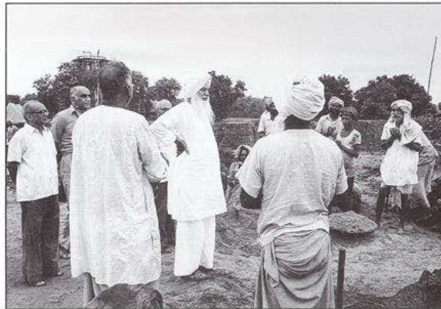
Maharaj Ji talking with sevadars at the construction site.
